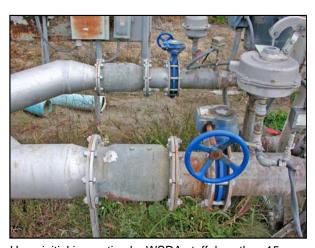
Upon initial inspection by WSDA staff, less than 15 percent of the irrigation systems used for chemigation or fertigation was deemed compliant. The above-pictured system lacked an inspection port, low-pressure drain, and vacuum relief valve, all required devices.
